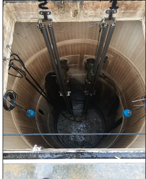
Photograph 7-7 Boeing Pump Station Wet Well
