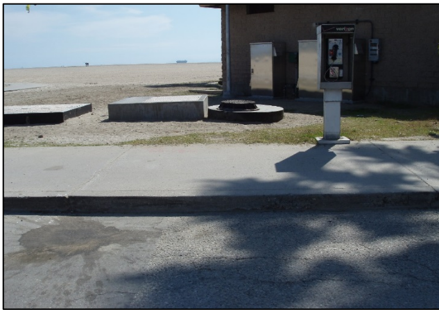
Photograph 7-10 1 st Street Pump Station Pump Station Site with 2007 Improvements
