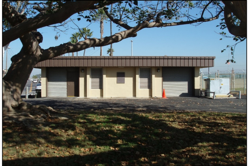
Photograph 7-14 Pump Station 35 Pump Station Housing
