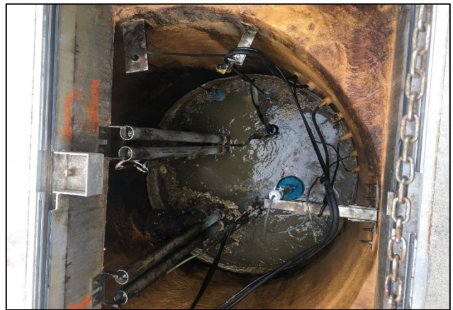
Photograph 7-11 1 st Street Pump Station Wet Well
