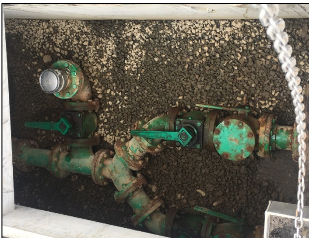
Photograph 7-12 1 st Street Pump Station Valve Vault
