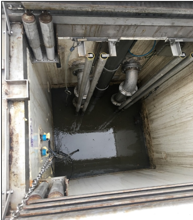
Photograph 7-8 8 th Street Pump Station Wet Well
